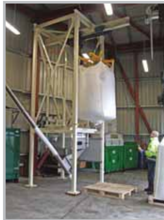
3. Traversing bag into position.
